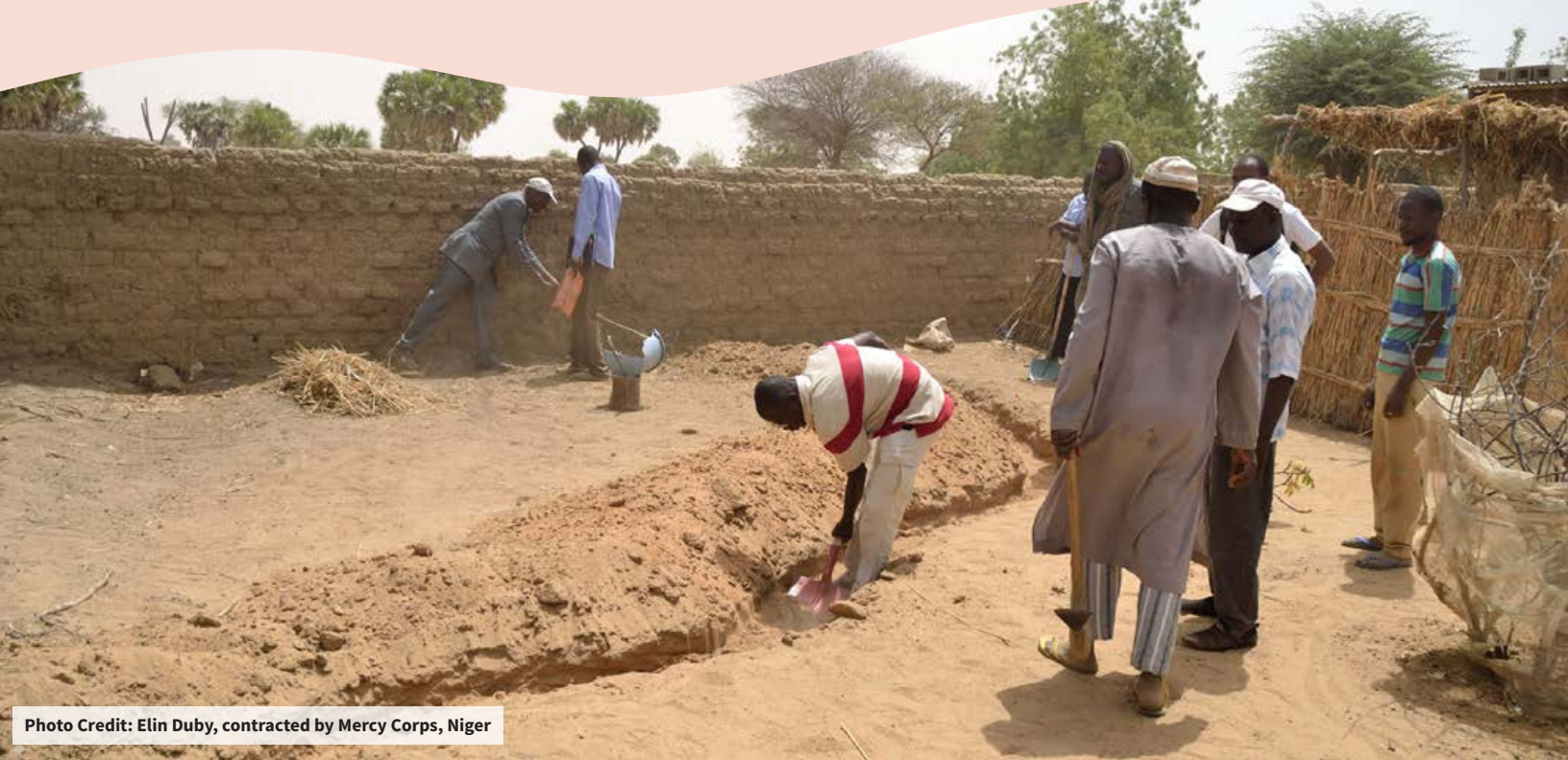
Digging an on-contour swale
