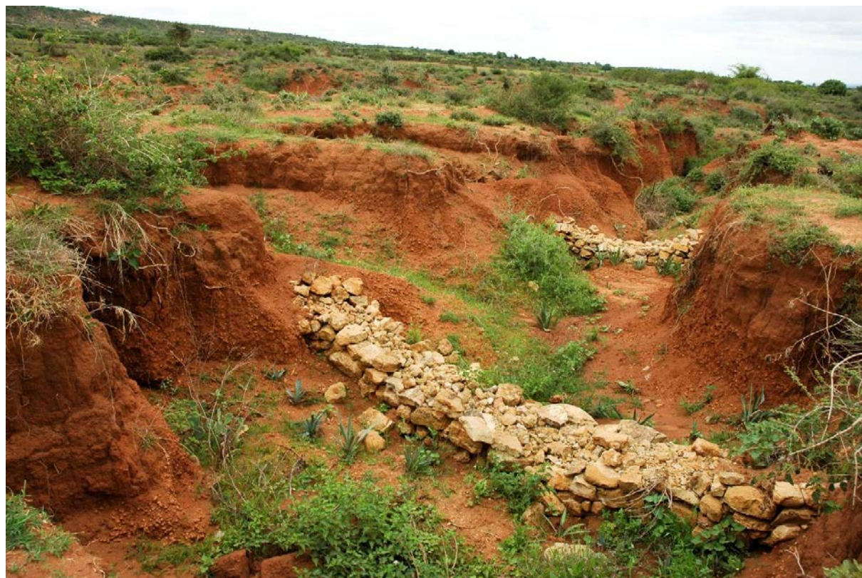
Rock check dams slowing water flow in Ethiopia.
