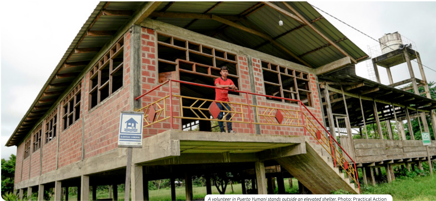
A volunteer in Puerto Yumani stands outside an elevated shelter. Photo: Practical Action
